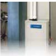
**A cased indoor coil is installed on top of a furnace.** A Micro-Channel coil is made of all aluminum. Eliminating copper helps the coil resist corrosion.
