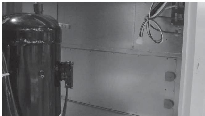
**Figure 4. Electric Heat Access Plate**
