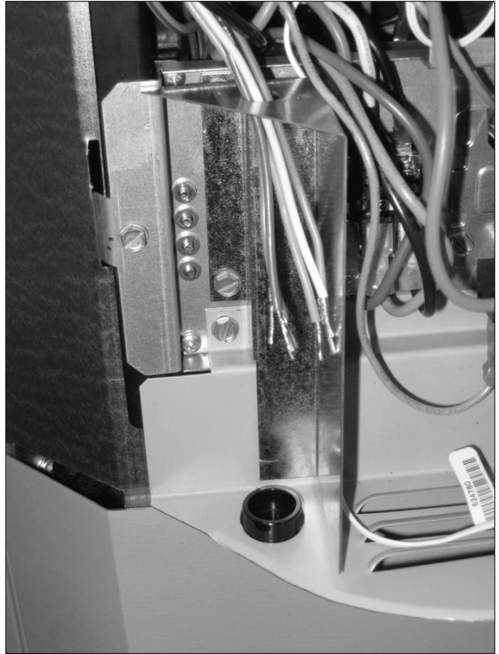
Figure 6. Low Voltage Compartment for Control Wiring
