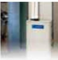
**A cased indoor coil is installed on top of a furnace.** An Anteater MC<sup>®</sup> Micro-Channel coil is made of all aluminum. Eliminating copper helps these coils resist formicary corrosion, the number one cause of coil leaks.
