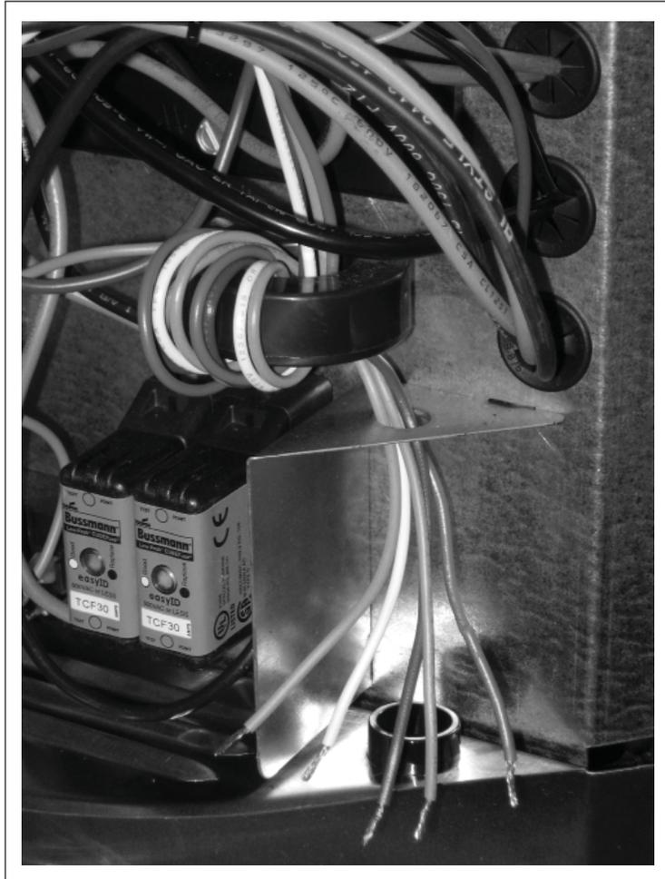
Figure 5. Low Voltage Control Wiring Compartment
