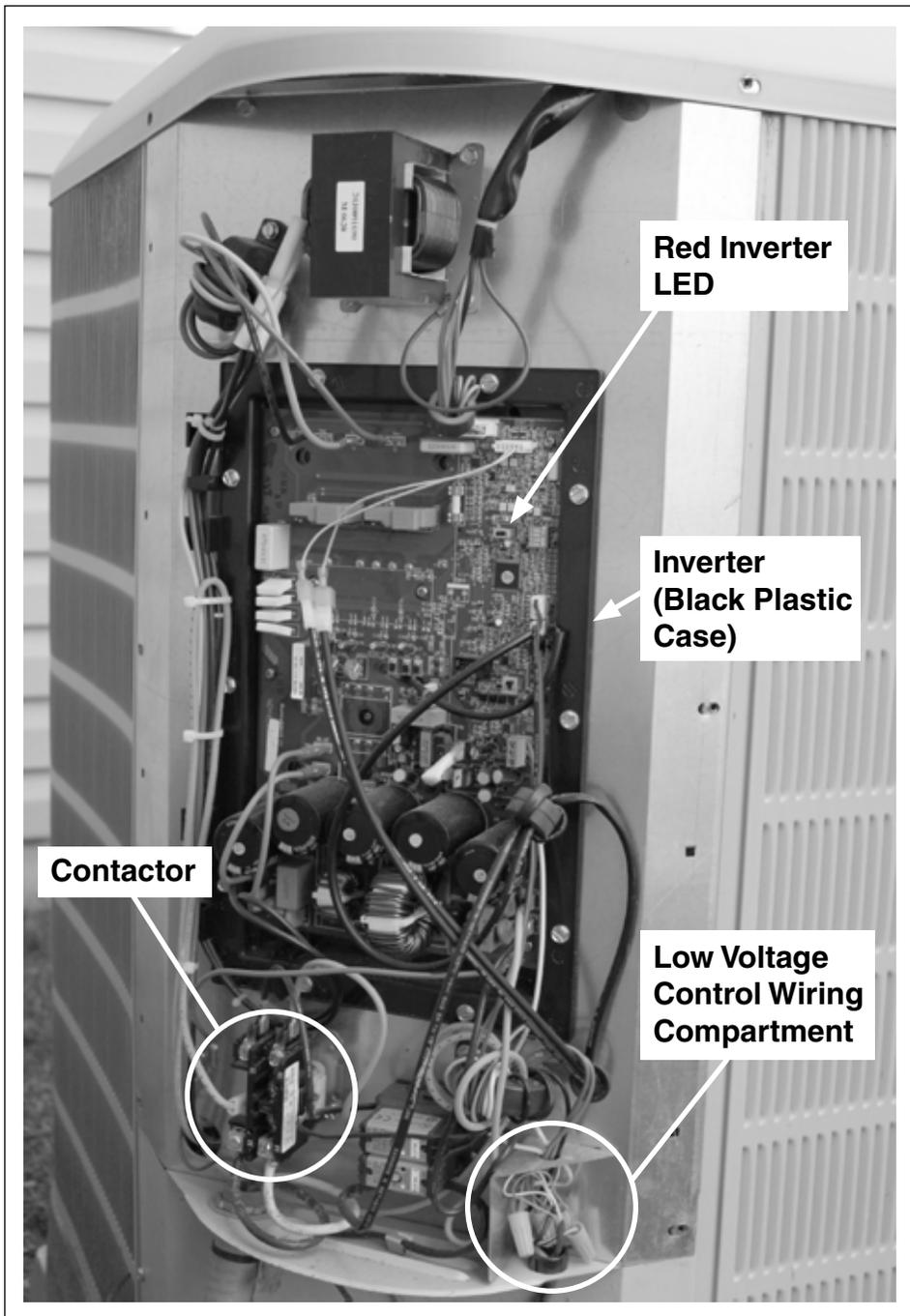
**Figure 3. iQ Drive Air Conditioning Control Panel**
